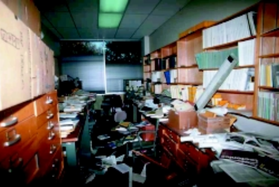
Books and air-conditioning duct were dislodged during Loma Prieta Earthquake. [J.K. Nakata, U.S. Geological Survey]
