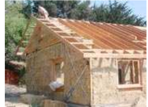
Placing final bales in gable end
