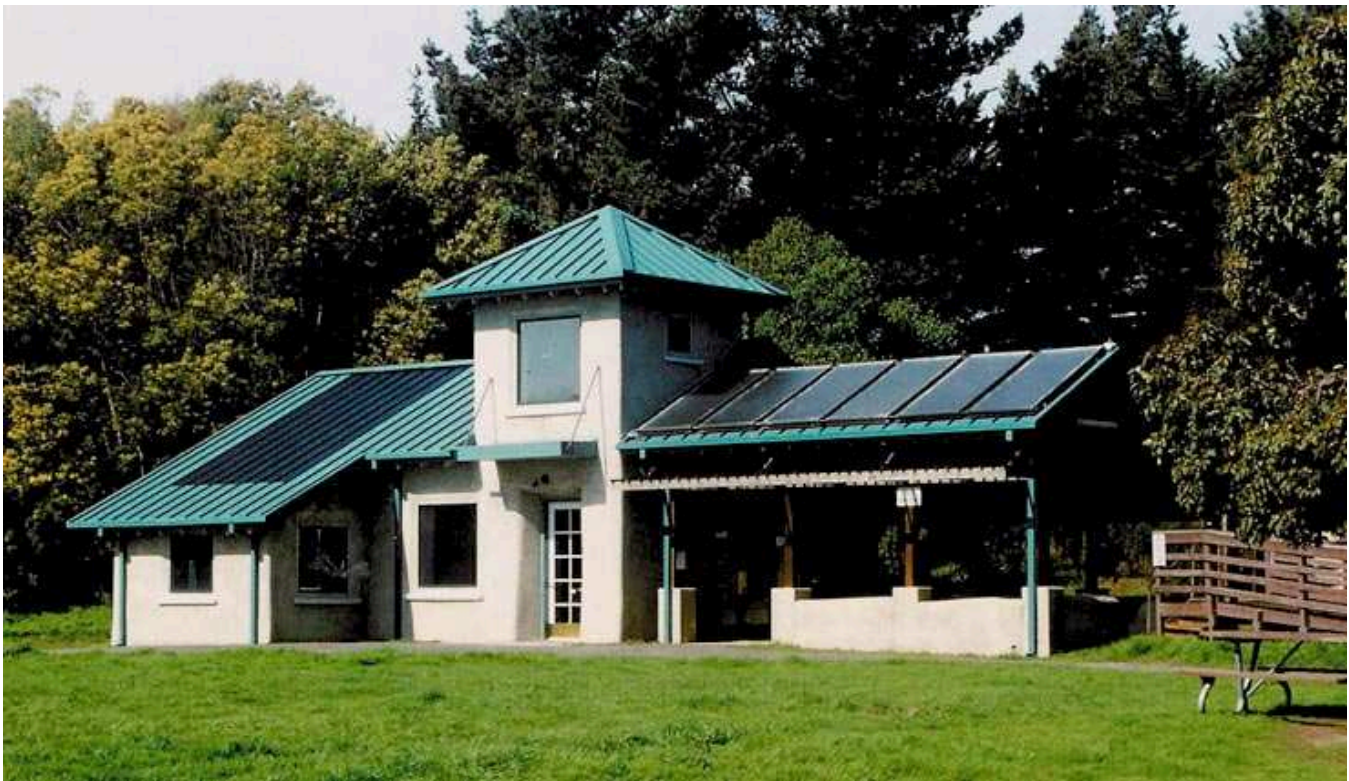
South View of the Nature Center. Photovoltaic panels are on the left roof, hot water solar panels are on the right roof.
