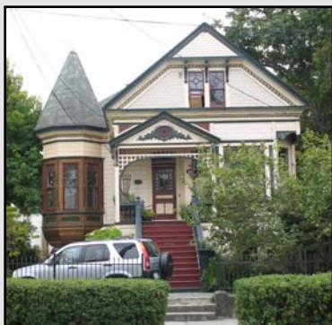
Image 59: 1940 Channing Way is an example of a Victorian residence in Downtown Berkeley (source: Nick Perry for ARG, August 2006).
