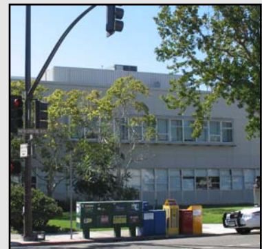
Image 53: The Alameda County Courthouse at 2120 Martin Luther King, Jr. Way (source: Nick Perry for ARG, August 2006).
