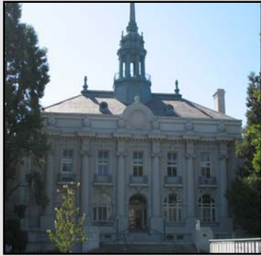
Image 44: A current view of the 1909 City Hall Building (source: Nick Perry for ARG, August 2006).
