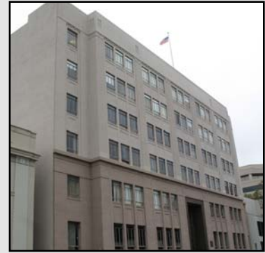
Image 52: The State Farm Building at 1947 Center Street (source: Nick Perry for ARG, August 2006).
