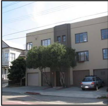
Image 77: 1915 Bonita Avenue (source: Nick Perry for ARG, August 2006).
